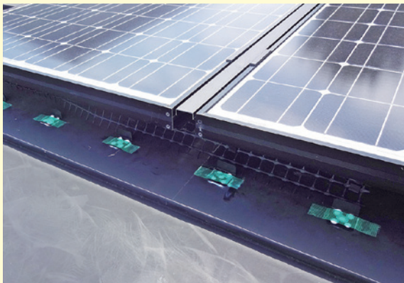
③固定金具の貼付
